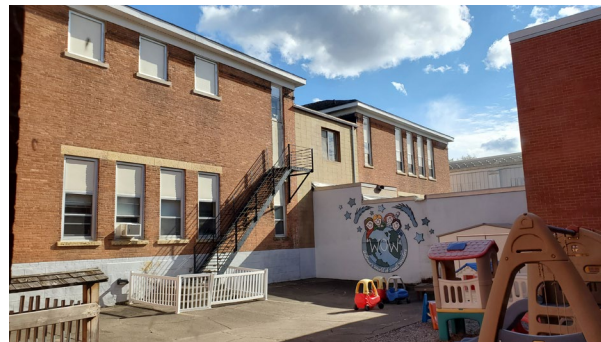
Fig. 12: 1973 infill structure with tan block between the 1870 and 1872 additions, and a one-story corridor connection to the 1960 addition.
