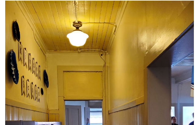
Incandescent lighting in an 1848 corridor.
