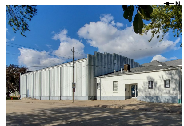
Fig. 10: The gymnasium in 2021 with the 1962 cafeteria addition.
