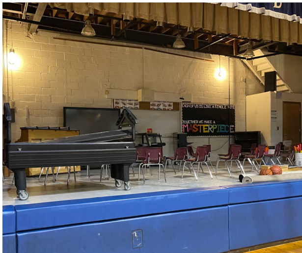
Fig. 11: The existing stage, currently being utilized as a music room, does not have an accessible ramp to allow wheelchair access.
