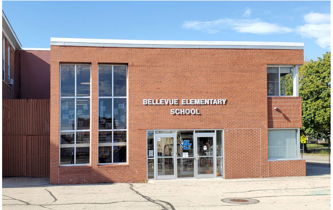
Fig. 15: The 2013 first floor administrative office renovation is slightly visible by variations in brickwork and brick joint lines. The 2005 elevator tower addition is visible in the background, tucked between the 1848 building and the 1973 addition.
