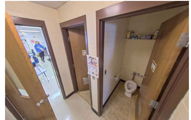
Fig. 19: Non-compliant single-use restrooms and hallway connecting two 1973 classrooms.
