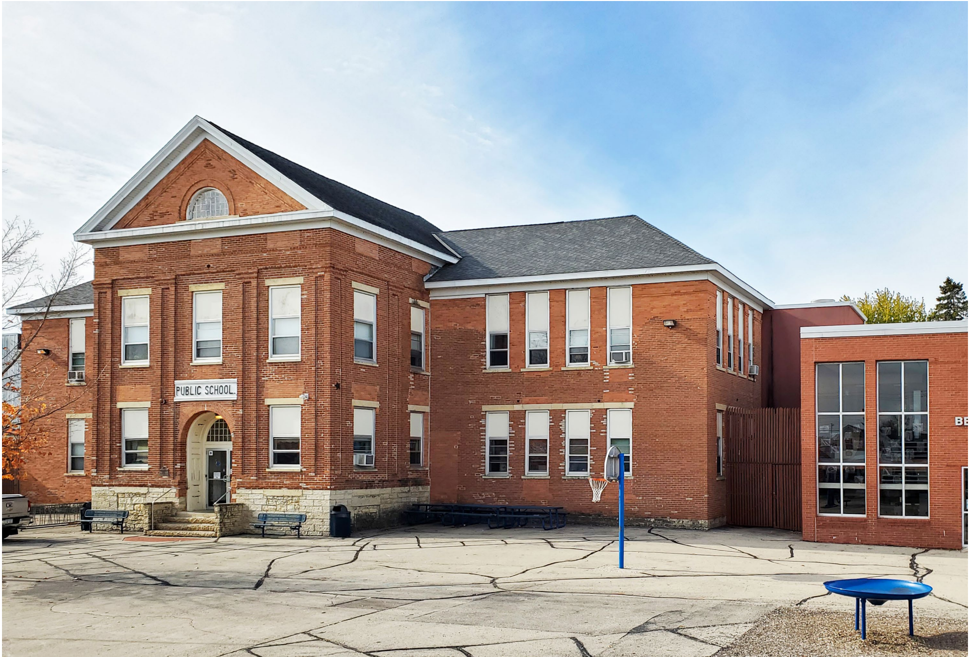
Fig. 6: Evidence that previous door and window openings from 1848 were removed or modified in the 1870s can be seen by variations in brick color. The north and south wings of the building also appear to have been raised several feet in height.
