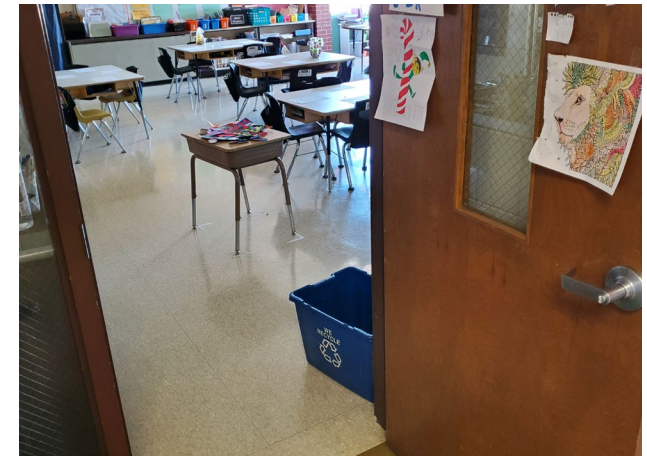
Fig. 8: Wire glass windows in the 1973 addition are no longer allowed by code due to the tendency to shatter and cause injuries.
