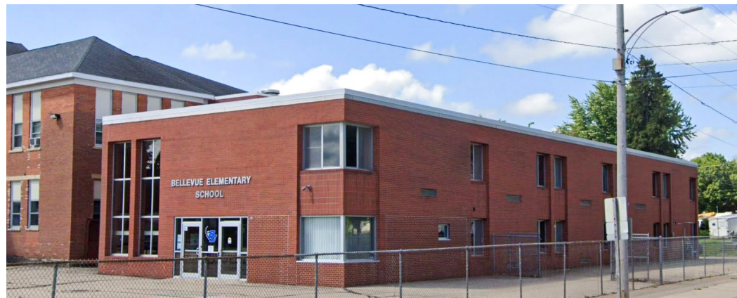
Fig. 13: The 1973 addition next to the 1848 original building. A remodel in 2013 converted the previous recessed entrance into a new administration office and secure entrance for the elementary school.
