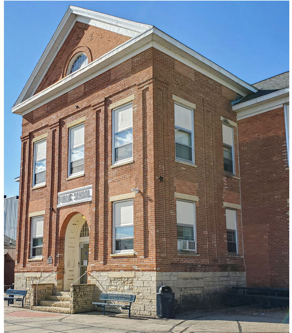
Fig. 1: Newer single-pane operable windows and older single-pane arched windows. Building cornices do not have gutters and allow water to drip onto wall surfaces, which is causing moisture issues at the base of the building.
