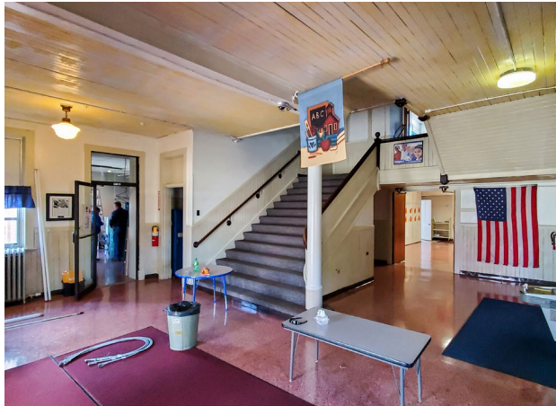
Fig. 7: The central stair in the 1848 building is open to adjacent spaces and does not have any fire separation between the basement and upper floors, creating a three-story space. No other stairs in this portion of the building are compliant with egress or fire separation.
